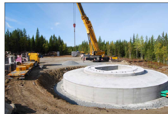
Fundament (foto: Jonas Lundmark)
